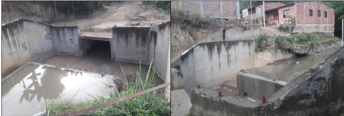
Box culvert Tierra Santa
